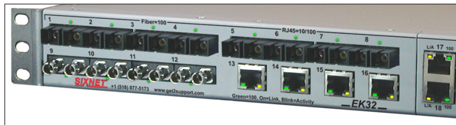
Ethernet Port Group 1
