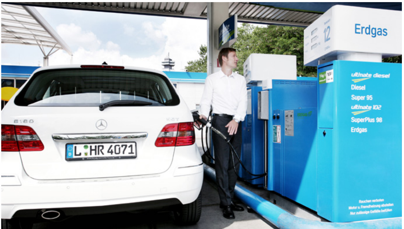
CNG fueling station
